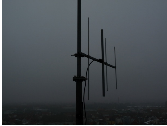
Figure 1: Transmitting antenna for vertical polarised transmission
